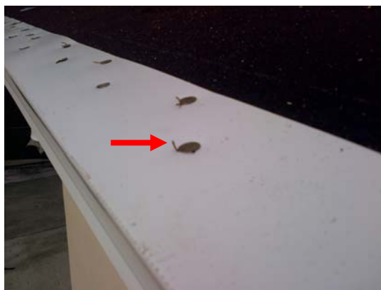
Residual metal "hair" at drip edge
