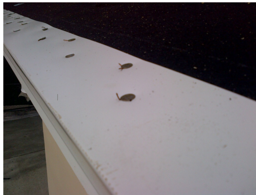
Figure 1: Residual metal “hair” at drip edge
