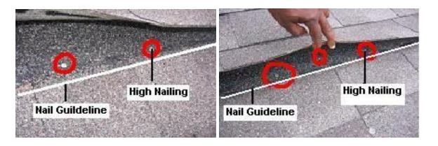
Note: Some premium shingles have different measurements or enhanced nailing areas. Be sure to check the installation instructions for correct placement of the nails prior to application.
