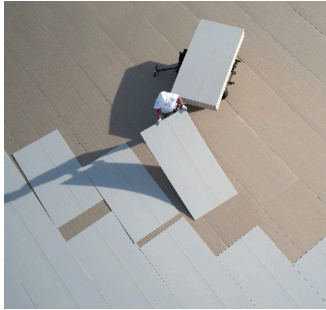
Image 2. HD polyiso cover board installation. Image courtesy of GAF.
