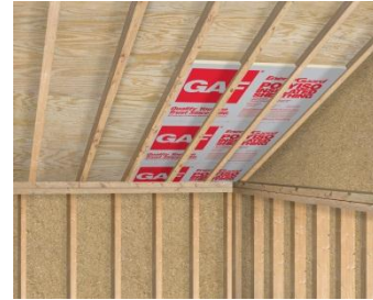
Vaulted Ceiling (Between joists)
