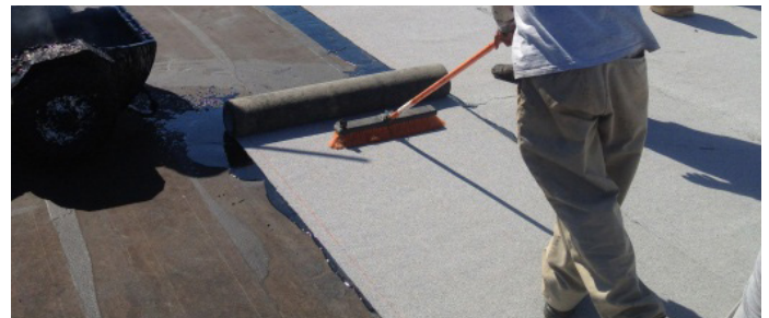
SBS modified bitumen rolls installed using a cold-applied adhesive.
