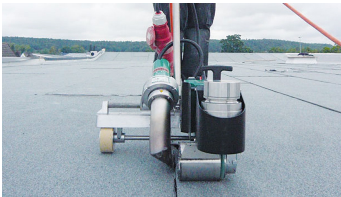
Sealing the seams of an SBS membrane with a welder, similar to the method used to seal seams of a single-ply membrane.
