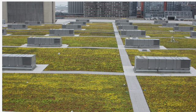
A vegetative low-slope roof.
