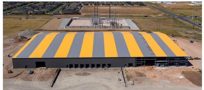
Austin Hose Headquarters, Amarillo, TX. Roofing System: EverGuard® TPO 60-mil Smooth Membrane in a custom Goldenrod yellow and Slate Gray design
