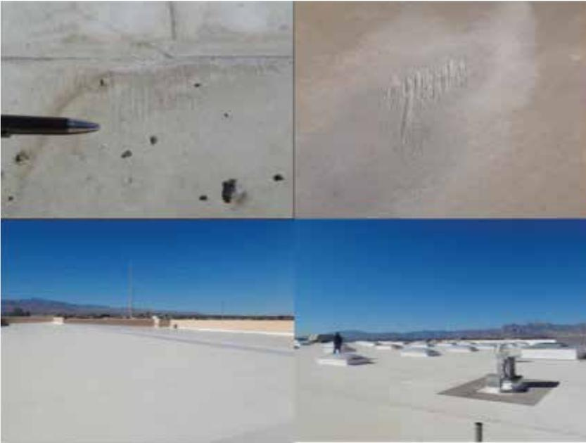
Clockwise from upper left: A five-year-old roof showing cracking; a seven-year-old membrane showing erosion to the scrim; a 10-year-old 60-mil membrane; and a 12-year-old 45-mil membrane. The latter two roof systems showed negligible signs of weathering and were located in Las Vegas.
