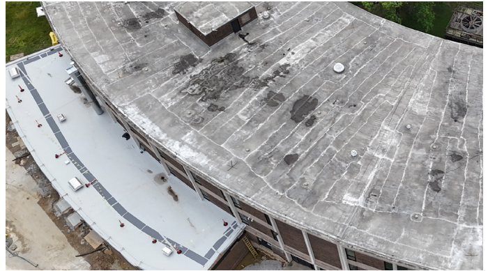
Classroom wing, before.
