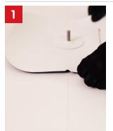
Align the GAF Rooftop Equipment Mount 240 according to the engineered design. Most designs are transferred to the roof surface with chalk lines. Guide notches can be used to align with the solar array layout to ensure an easier and accurate installation.
