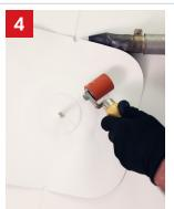
Hot-air-weld the perimeter edge of the cover membrane using a 2-inch roller to achieve a minimum 2-inch weld around the perimeter. Probe the seam to make sure the membrane is welded properly.
