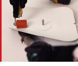
For use with TPO and PVC membranes.\* The location and number of mounts in addition to the number of fasteners per mount shall be determined by the project design professional to resist the calculated pressures. The following instructions are meant to be utilized by an experienced and professional roofing contractor using the proper equipment, techniques, and safety protocols.
