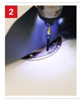
Install the GAF Rooftop Equipment Mount 240 using the correct type and quantity of fasteners specified by your design professional.
