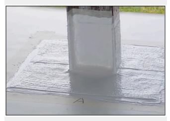
7. Top coat the embedded GAF PMMA Fleece with an 8. additional layer of GAF PMMA Flashing resin.
