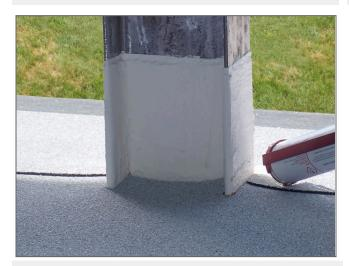
11. Apply a bead of GAF M-BOND<sup>TM</sup> Adhesive Sealant around the base of the penetration to fill any gaps between the SBS roof membrane system and the penetration.
