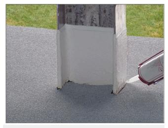
11. Apply a bead of GAF M-BOND<sup>™</sup> Adhesive Sealant around the base of the penetration to fill any gaps between the SBS roof membrane system and the penetration.
