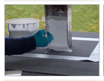
Mix the GAF PMMA Catalyst and GAF PMMA Flashing as detailed in the mixing instructions. Apply a base coat of GAF PMMA Flashing to the vertical penetration surfaces extending onto the smooth ply a minimum of 2 in. 4. Apply the pre-cut GAF PMMA Fleece to the vertical penetration surfaces by embedding the fleece in the flashing, extending the fleece a minimum of 2 in. onto the roof membrane. Ensure that no air is trapped beneath the fleece.
