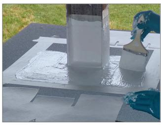
6. Apply a base coat of GAF PMMA Flashing to the horizontal surface extending to the masking tape. Apply the pre-cut GAF PMMA Fleece to the horizontal surface by embedding the fleece in the GAF PMMA flashing. Saturate all fleece surfaces to be lapped with GAF PMMA Flashing. Pieces of fleece must overlap by at least 2 in. (50 mm).
