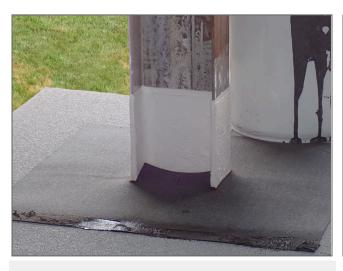
After the flashing is set, a target of smooth ply material is applied over the finished GAF PMMA Flashing membrane. Extend the target a minimum of 4 in. beyond the GAF PMMA Flashing membrane in all directions.
