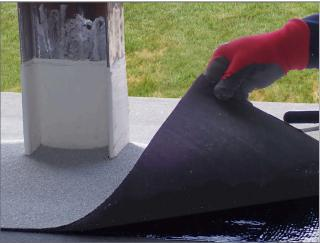
After the flashing is set, a target of base ply material is applied over the finished GAF PMMA Flashing membrane. Extend the target a minimum of 4 in. beyond the GAF PMMA Flashing membrane in all directions.
