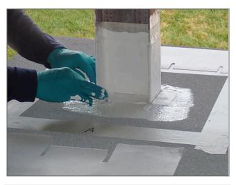
5. Apply the pre-cut GAF PMMA Fleece to the vertical penetration surfaces by embedding the fleece in the GAF PMMA flashing, extending the fleece a minimum of 2 in. onto the roof membrane.
