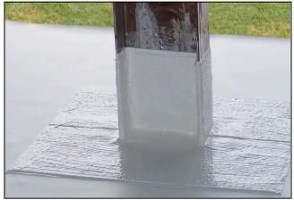
8. Remove the masking/painter's tape before the flashing sets completely.
