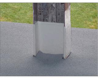
Apply a target of granulated surface membrane, ensuring that it fits tightly around the penetration.
