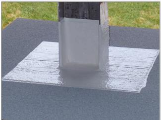
Remove the masking/painter's tape before the GAF PMMA flashing sets completely.
