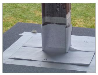
3. Cut the GAF PMMA Fleece for the penetration configuration, extending 6 in. up the penetration and 6 in. out onto the horizontal. The pieces of fleece must overlap by at least 2 in. (50 mm). Place each piece dry in its designated area to ensure proper fit and laps. Install masking/painter's tape a maximum 1/4 in. beyond the edge of the GAF PMMA Fleece, both on the top of the penetration and the horizontal surface.
