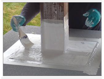
7. Top coat the embedded GAF PMMA Fleece with an additional layer of GAF PMMA Flashing. The GAF PMMA Fleece must be sufficiently coated with the GAF PMMA Flashing to prevent the GAF PMMA Fleece from telegraphing through.
