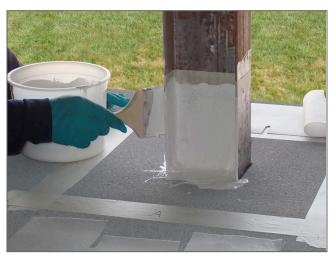
4. Mix the GAF PMMA Flashing with the GAF PMMA Catalyst as detailed in the mixing instructions. Apply a base coat of GAF PMMA Flashing to the vertical penetration surfaces, extending onto the roof membrane a minimum of 2 in.
