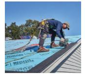
Installs at the eaves and rakes to reduce the risk of shingle blow-off
