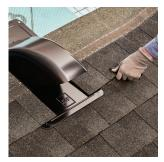
Shingles are run over the top and sides of the base flashing and cut around the hood for a clean, finished look
