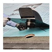
5.5" (140 mm) diameter circular opening cut in roof deck with included template on packaging
