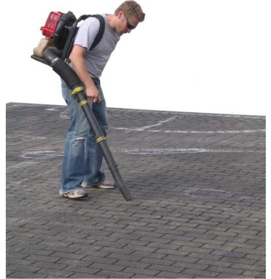
**Important! StreetBond® Coatings are meant to adhere to the oils in the asphalt pavement. If there is a contaminant on the surface, it may affect adhesion.**
