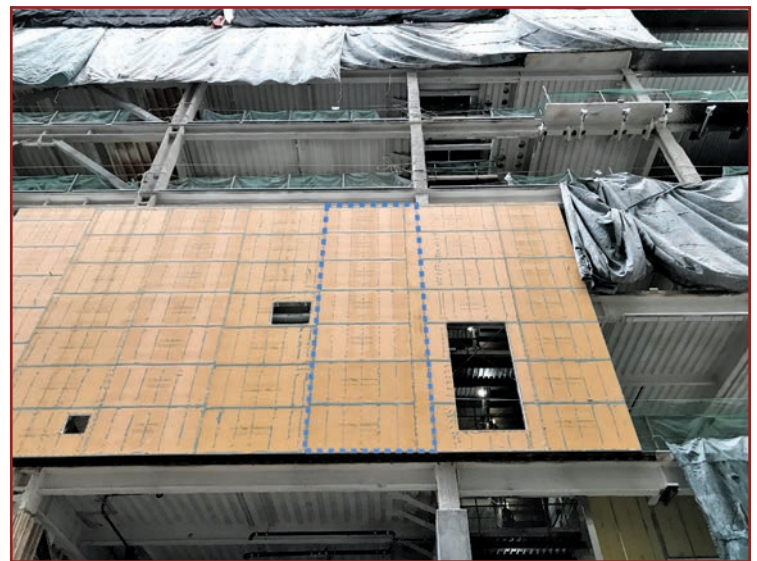
Figure 5. Large-format panels on a commercial high-rise building. Panel size is indicated by the blue dashed lines.
