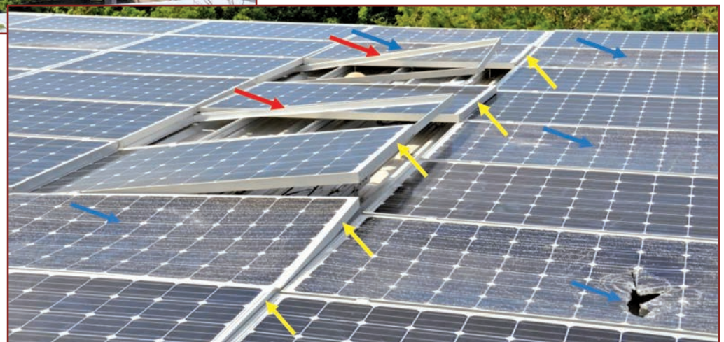
Figure 32. The red lines indicate where several adjacent solar panels were blown off during Hurricane Irma (US Virgin Islands, 2017). The area within the red oval in the left photo is the focus of the right photo, where the red arrows indicate the polyvinyl film detached from the panel frame. Some panels lifted but did not blow away (yellow arrows). Some panels were damaged by wind-borne debris (blue arrows). Source: Federal Emergency Management Agency. 25
