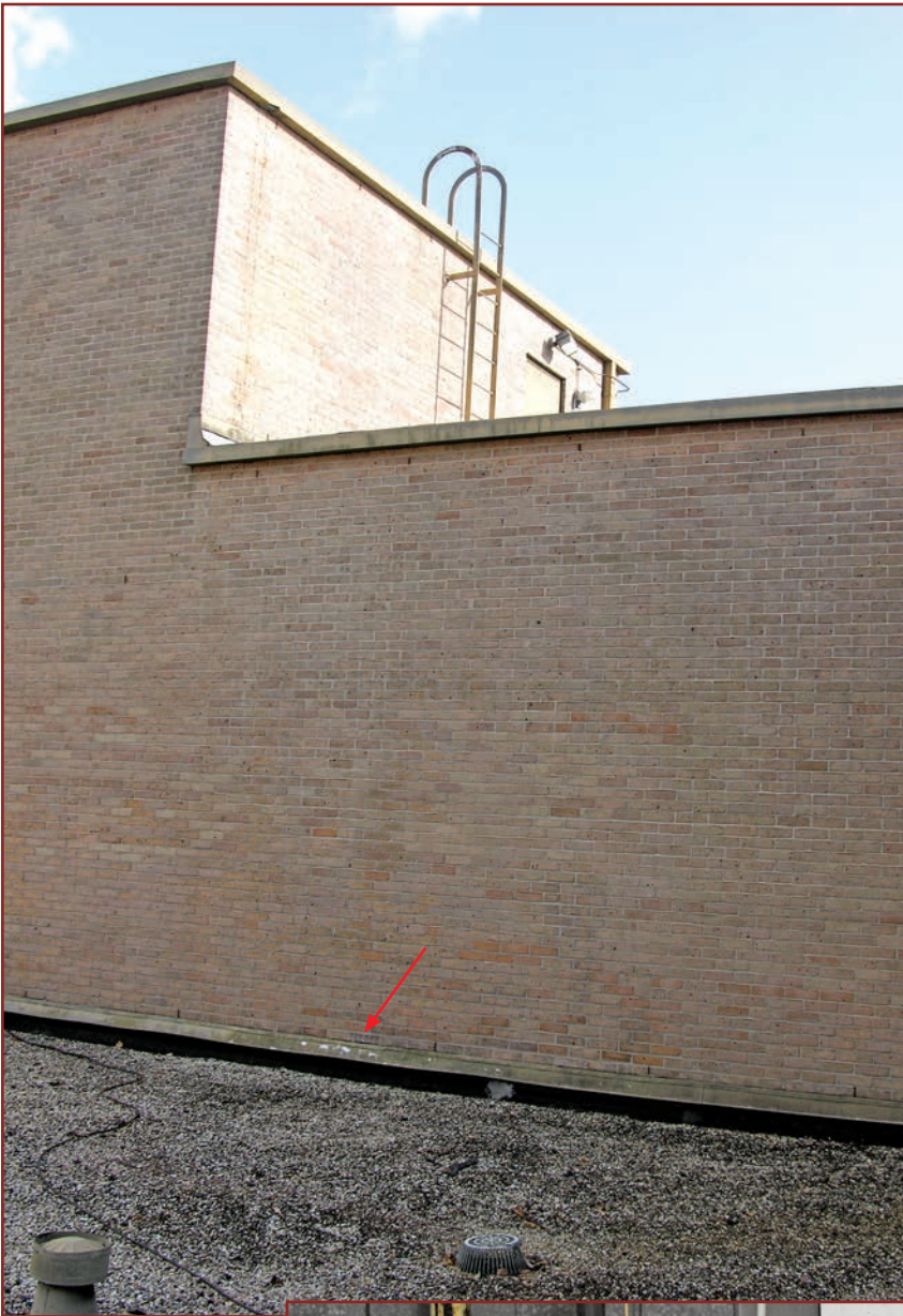
Figure 17. At this Louisiana hospital, water leaked into the building along the base of many of the brick veneer walls during Hurricane Katrina (2005). It was believed that rain was blown into the wall cavity, where it overwhelmed the capacity of the weeps and inundated the through-wall flashings. Source: Federal Emergency Management Agency (FEMA 577). 20
