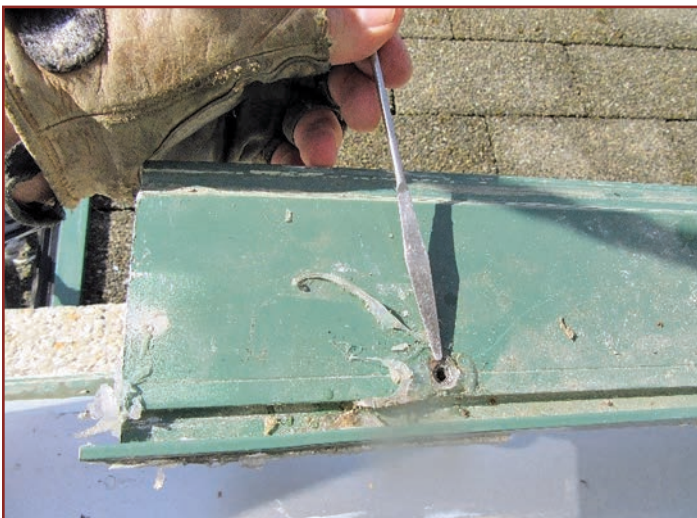
Figure 3. Fastener penetration through a subsill.
