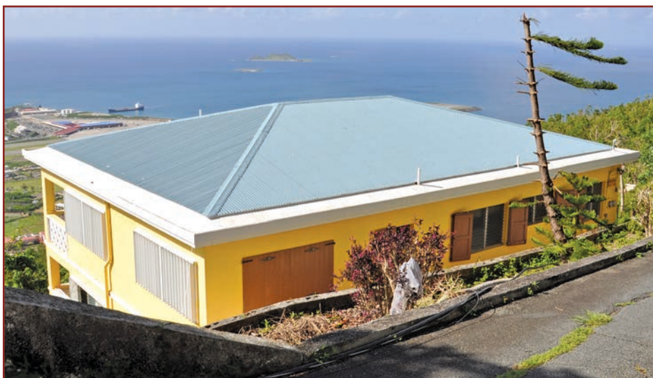
Figure 33. During Hurricane Irma (US Virgin Islands, 2017), there was no apparent damage to this building enclosure (the interior was not evaluated for entrance of wind-driven rain). The estimated wind speed was approximately 175 mph (including wind speed-up due to an abrupt change in topography). Source: Federal Emergency Management Agency (FEMA P-2021). 57
