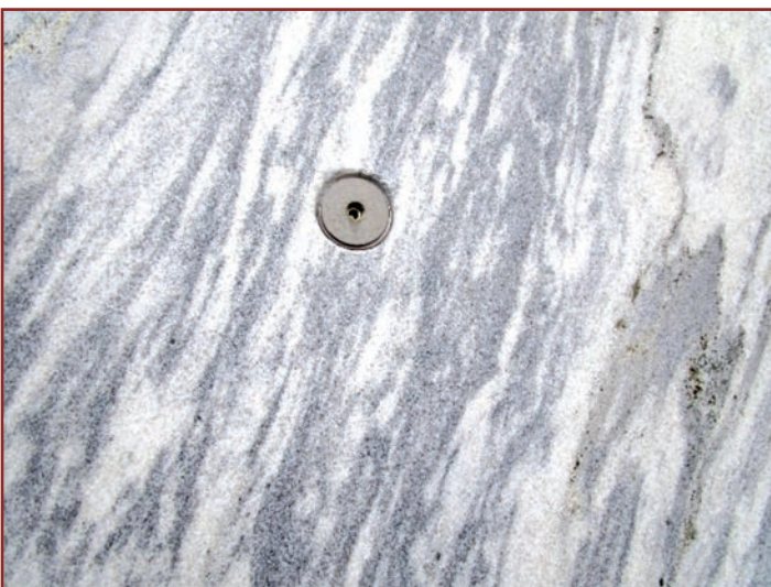
Figure 10. Installed custom stone anchor into the marble cladding (left) and torque testing (right).
