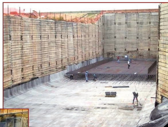
Figure 4. Mat slab under construction.
