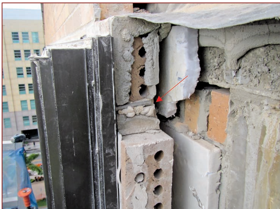
Figure 14. Hurricane shutter anchorage was not attached to structure.
