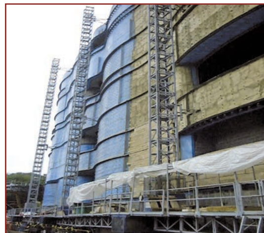
Figure 4. Air barrier system for six sides of the building.
