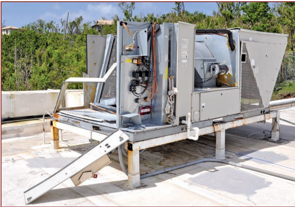
Figure 31. The sheet metal enclosure (cabinet) blew off this heating, ventilation, and air-conditioning unit during Hurricane Irma (US Virgin Islands, 2017). An access panel was also blown off. It appeared that wind-blown enclosure debris caused roof membrane tears. Source: Federal Emergency Management Agency (FEMA P-2021). 57
