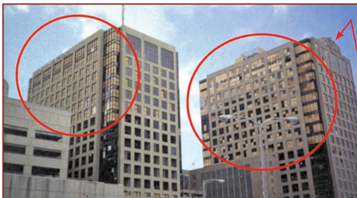
Figure 8. Most of the glazing in the red circles was broken by built-up roof aggregate. Further information on the glazing damage is given in Crandell and Smith. 10 This damage is reminiscent of glazing damage in the Houston, Texas, central business district during Hurricane Alicia (1993). The building on the right had a steep-slope roof; most of the mechanically attached single-ply membrane blew off. Estimated wind speeds were 145 to 170 mph.
