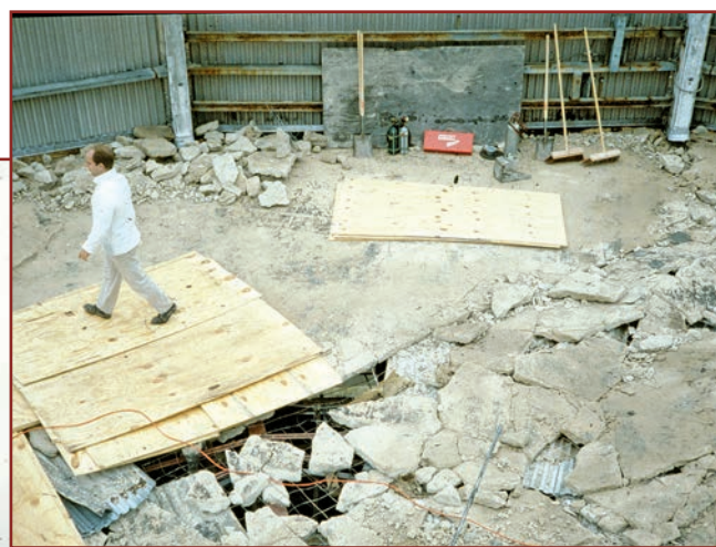
Figure 5. Roof deck damage (inset photo) at a midrise building. The estimated wind speed was around 100 mph. Source: Institute for Disaster Research, Texas Tech University. 7
