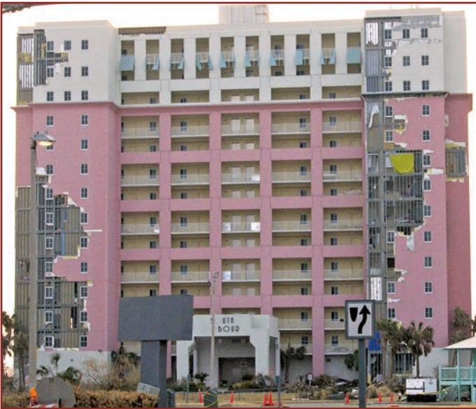
Figure 25. Damage that occurred during Hurricane Ivan (Alabama, 2004) to an exterior insulation and finish system (EIFS) at a residential building. The gypsum board typically detached from the studs. In some areas, the interior gypsum board was also blown off. EIFS can perform well, but wind damage is common. (EIFS damage also occurred at the hospital shown in Fig. 2.) Use of precast concrete wall panels would be a conservative design enhancement. Source: Federal Emergency Management Agency (FEMA 489). 52
