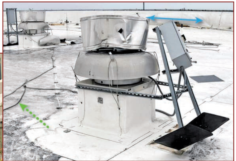
Figure 28. The fan in the foreground was struck by wind-borne debris. The fan's disconnect switch bracket was not adequately anchored. The green dotted arrow indicates a detached lightning protection system conductor. The blue arrow indicates detached base flashing. This damage occurred at the Florida hospital shown at Fig. 2 during Hurricane Michael (2018). Source: Federal Emergency Management Agency (FEMA P-2077). 1
