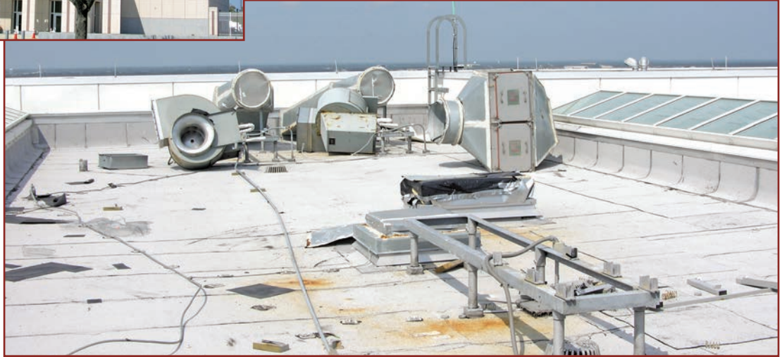
Figure 12. The rooftop equipment on this new federal courthouse in Mississippi blew away during Hurricane Katrina (2005) because fans were resting on vibration isolators that provided lateral resistance but no uplift resistance. Two large openings through the roof were left after the ducts blew away. The resulting water infiltration caused extensive interior damage. The building was not occupied for several months while repairs were underway. Source: Federal Emergency Management Agency (FEMA 543). 3
