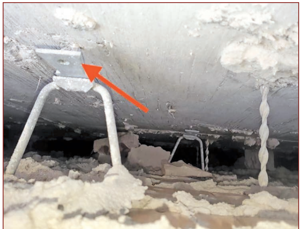
Figure 13. Detached existing brick ties and unengaged helical ties observed at one wall section.
