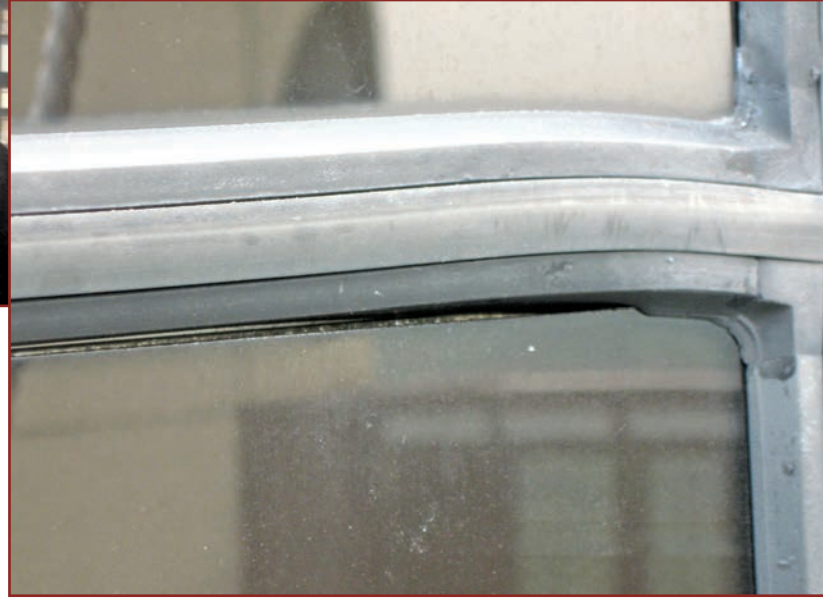
Figure 4. Dislodged glass below a floor line in an early curtainwall.
