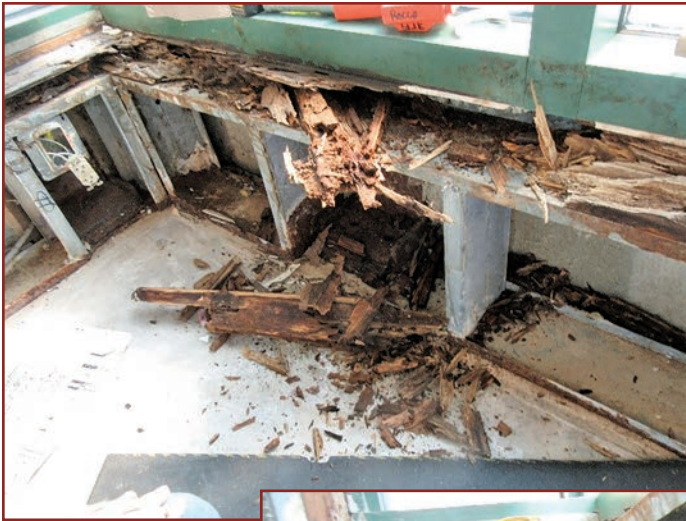
Figure 1. Decaying wood below a window frame.
