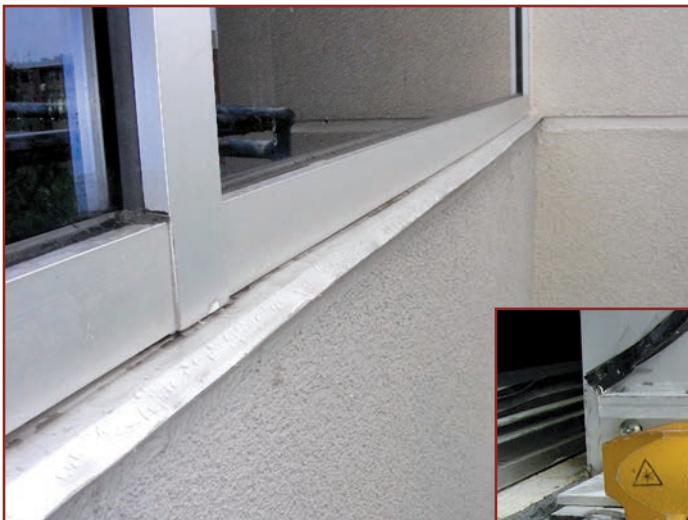
Figure 9. The drip edge of a pan exposed at the exterior.
