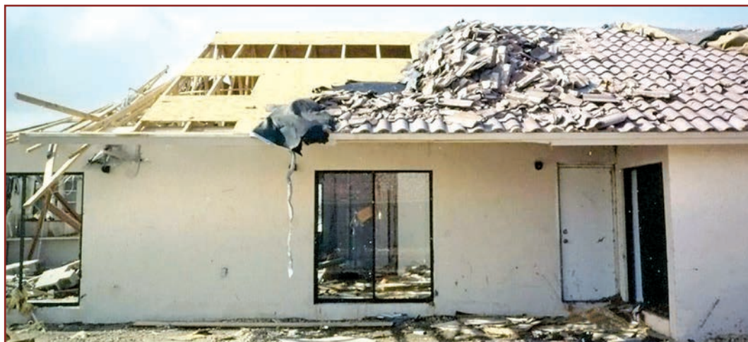
Figure 7. Poor structural performance overshadowed the performance of the building enclosure.
