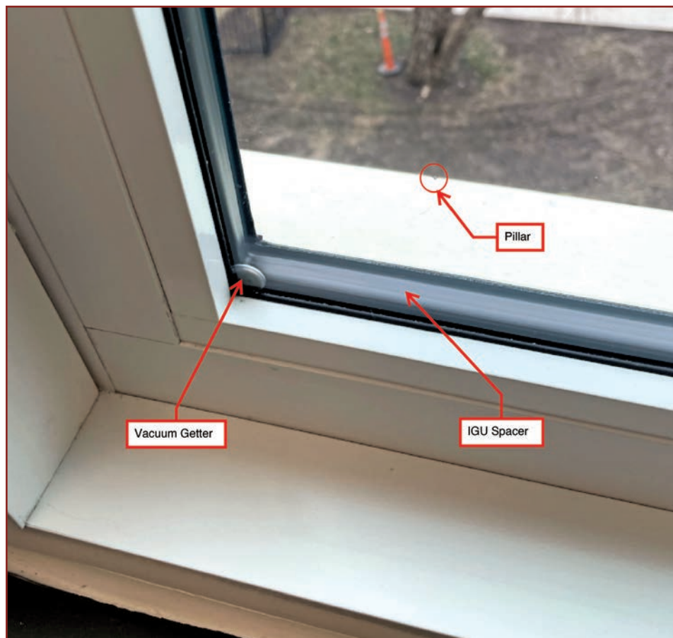
Figure 6. A corner of a hybrid-vacuum-insulated glass unit. Note: IGU = insulating glass unit.
