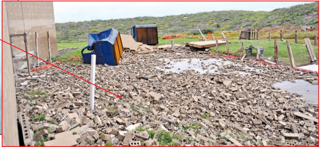
Figure 29. Brick veneer failure at a 12-story Texas condominium during Hurricane Harvey (2017). Before the storm, repairs had been made in the failed area using helical ties. The ASCE 7-16 2 basic wind speed for this building is 149 mph. The estimated wind speed was 140 mph (94% of the basic speed). Source: Federal Emergency Management Agency (FEMA P-2022). 40
