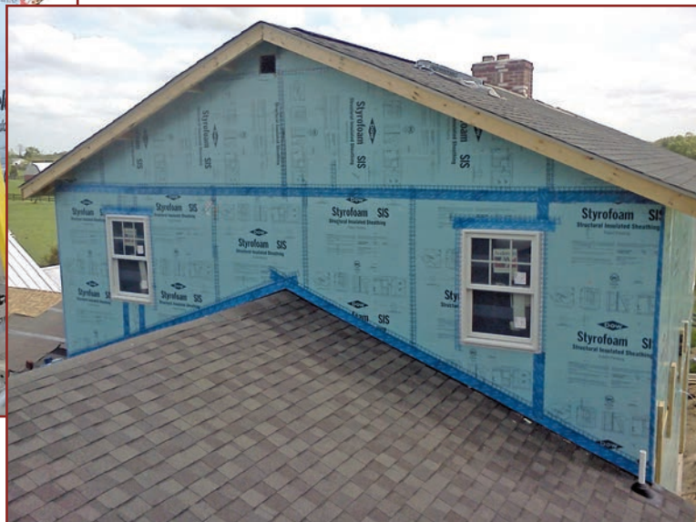
Figure 4. Adhered flashing and joint tapes used for foam plastic insulating sheathing water-resistive barrier systems and window flashing.
