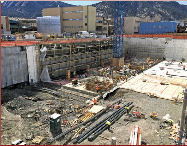
Figure 13. View of the preapplied sheet waterproofing being installed over the support of an excavation wall at a zero-lot line condition.
