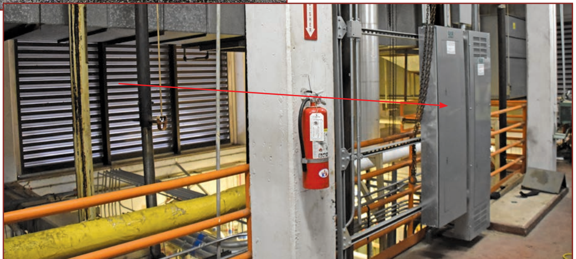
Figure 18. Although the estimated wind speed at this Florida hospital was only 115 mph, rain was driven several feet past the louvers and wetted the electric panels, which caused the circuit breakers to trip. Source: Federal Emergency Management Agency (FEMA P-2077). 1
