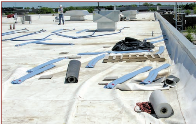
Figure 3. Detached roof membrane on a new police station in the Midwest. The winds were well below the basic wind speed. Source: Federal Emergency Management Agency (FEMA P-2062). 4
