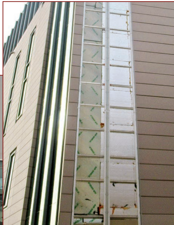
Figure 5. Terra-cotta rain screen veneer over continuous insulation.
