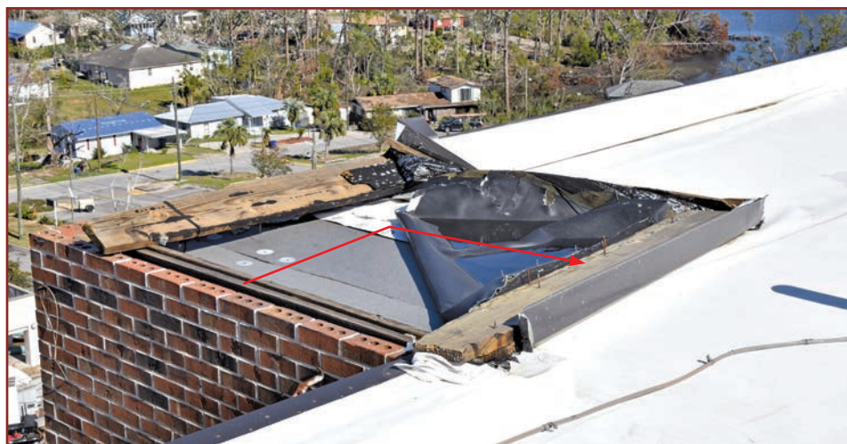
Figure 24. During Hurricane Michael (Florida, 2018), the nailer lifted and caused progressive lifting and peeling of the roof membrane. The ASCE 7-16 2 basic wind speed for this building is 147 mph. Estimated wind speed was 130 mph (88% of the basic speed). Source: Federal Emergency Management Agency (FEMA P-2021). 1
