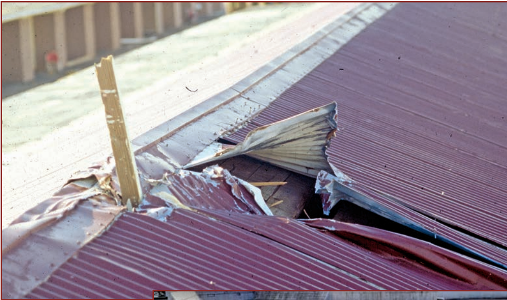
Figure 19. During Hurricane Marilyn (1995), a piece of 2x4 lumber penetrated the metal roof panel and 1x wood deck at a school in the US Virgin Islands. Source: Federal Emergency Management Agency Hazard Mitigation Technical Assistance Program.
