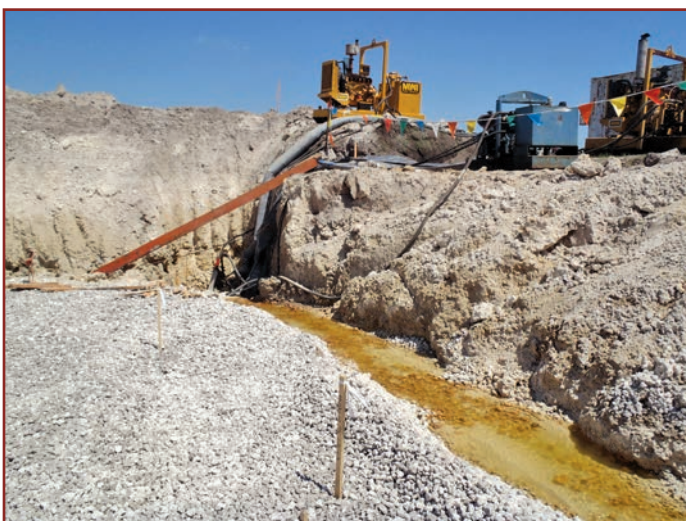
Figure 8. A dewatering pump station at a perimeter trench at the corner of the building pad.
