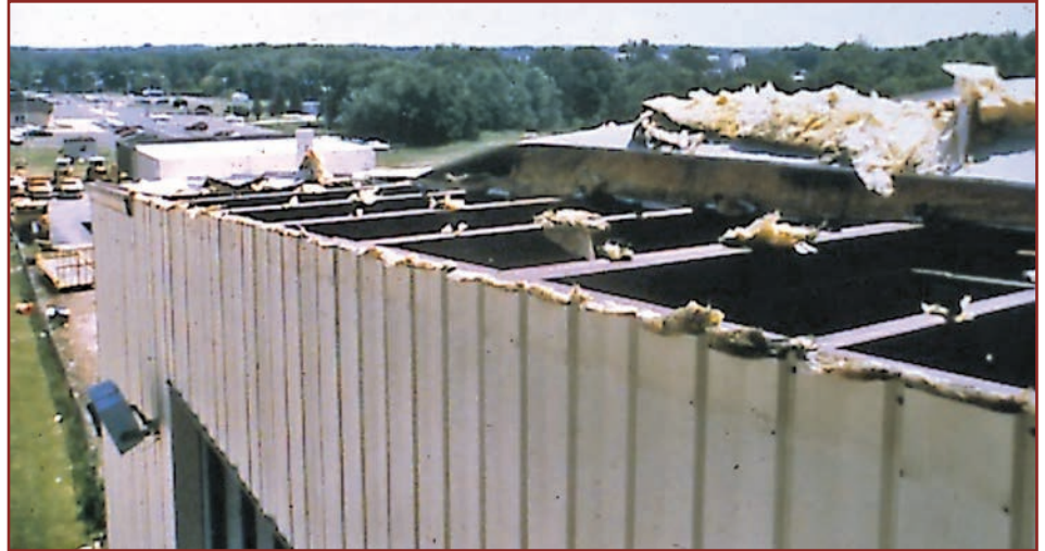
Figure 1. Typical wind failure of a standing seam roof.
