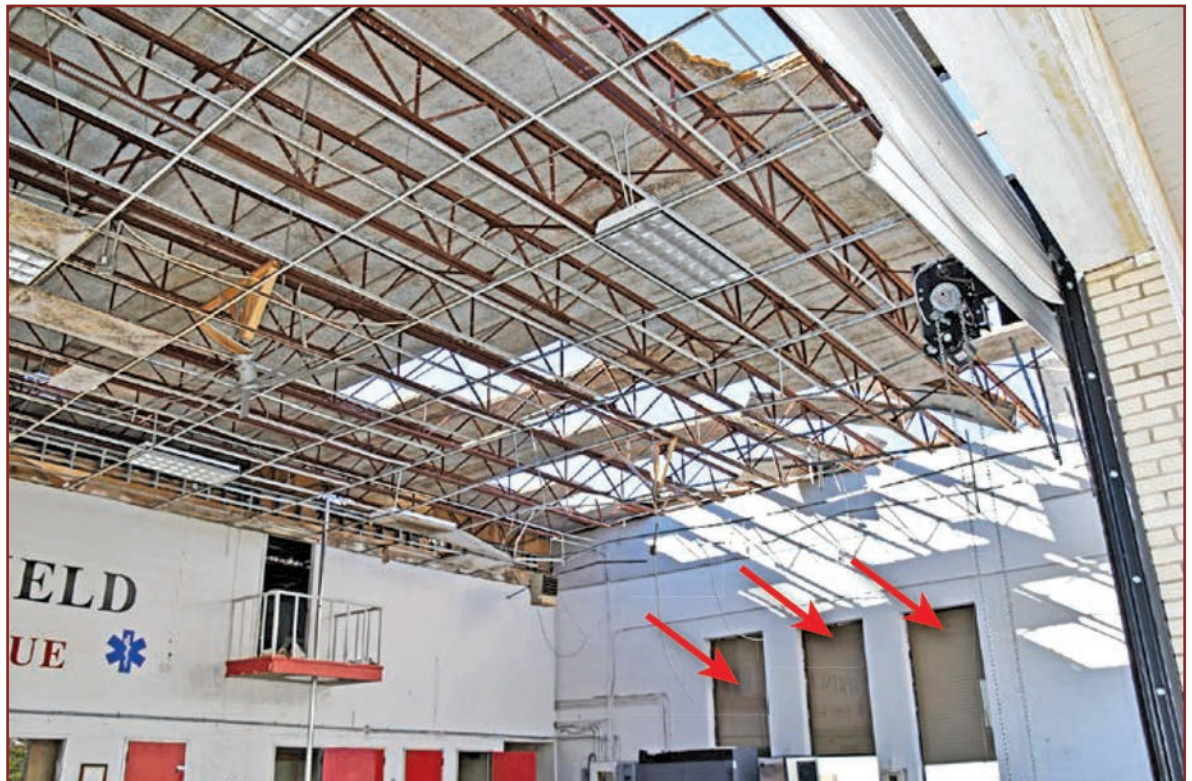
Figure 21. This Florida fire station was constructed in 1978. Around 2001, it was retrofitted with storm shutters (red arrows) and new apparatus bay doors (which failed during Hurricane Michael in 2018). These mitigations were unsuccessful because several of the cementitious wood-fiber deck panels blew off. The fire station was demolished after the storm. The ASCE 7-16 2 basic wind speed for this building is 146 mph. Estimated wind speed was 132 mph (90% of the basic speed). Source: Federal Emergency Management Agency. 46
