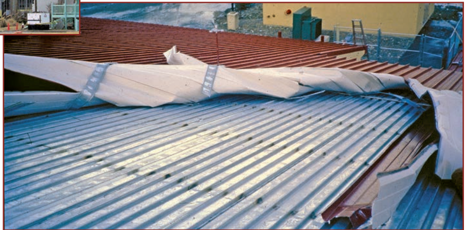
Figure 26. In the mid-1980s, the roof on this new school in Anchorage, Alaska, blew off during moderate winds soon after it was installed. It failed even though it was a robust system because of a major installation error.
