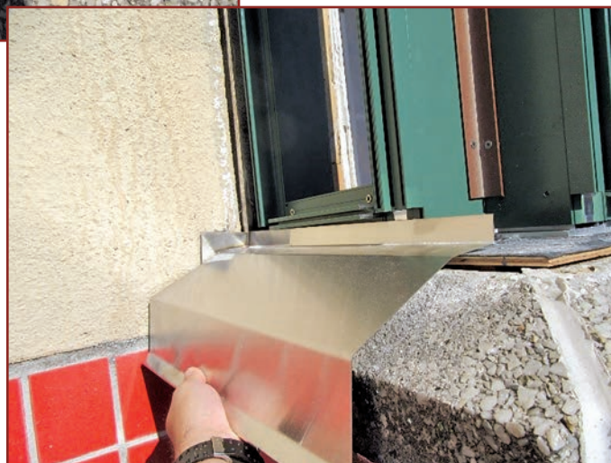
Figure 19. Supplemental flashing set into a glazing pocket under the mullion tongue.
