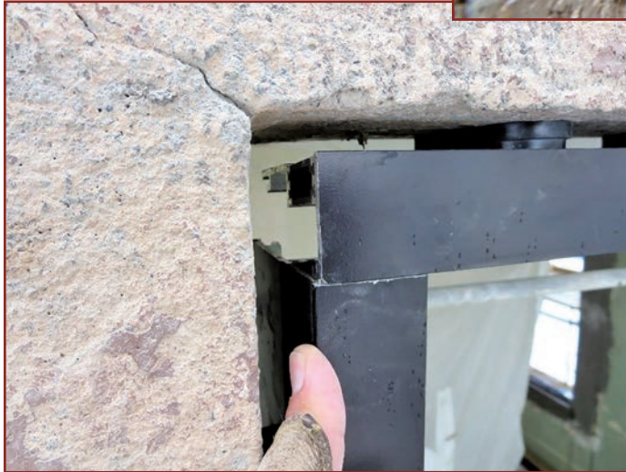
Figure 12. A gap between head and jamb frame components.
