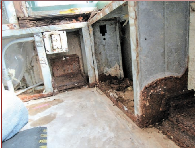
Figure 2. Corrosion of metal track and studs.
