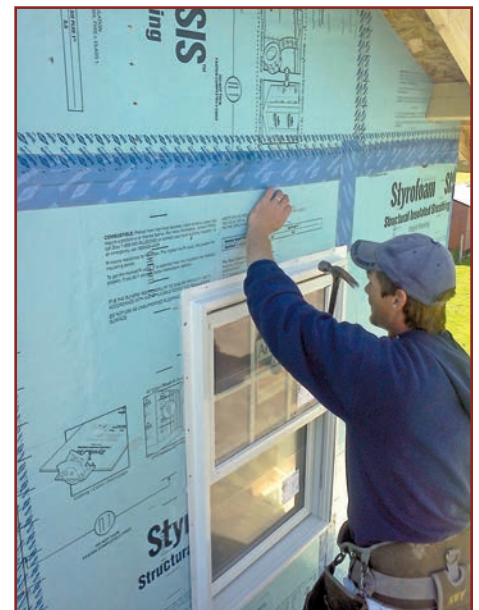
Figure 3. Typical installation of a flanged window directly over foam plastic insulating sheathing on a wood-frame home.
