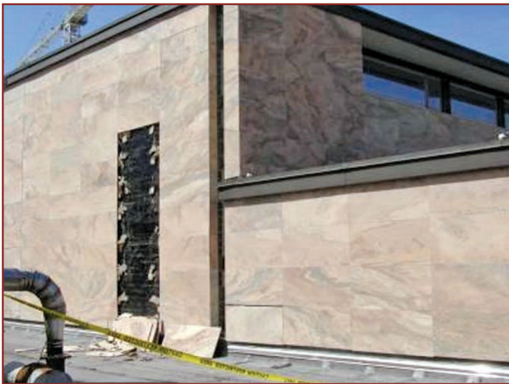
Figure 17. Area of panel detachment.
