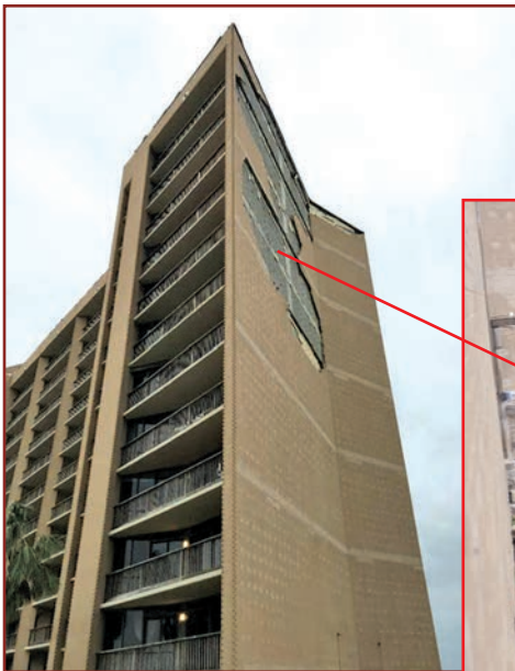
Figure 29. Brick veneer failure at a 12-story Texas condominium during Hurricane Harvey (2017). Before the storm, repairs had been made in the failed area using helical ties. The ASCE 7-16 2 basic wind speed for this building is 149 mph. The estimated wind speed was 140 mph (94% of the basic speed). Source: Federal Emergency Management Agency (FEMA P-2022). 40
