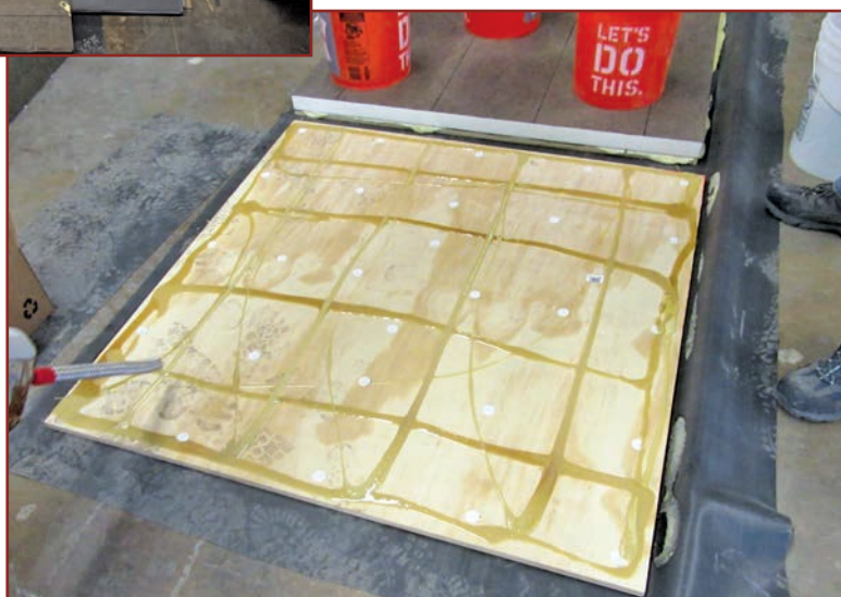
Figure 2. Grid of low-rise foam adhesive being applied to plywood panels to achieve an approximate 6 in. grid onto which one of the insulation boards would be placed.
