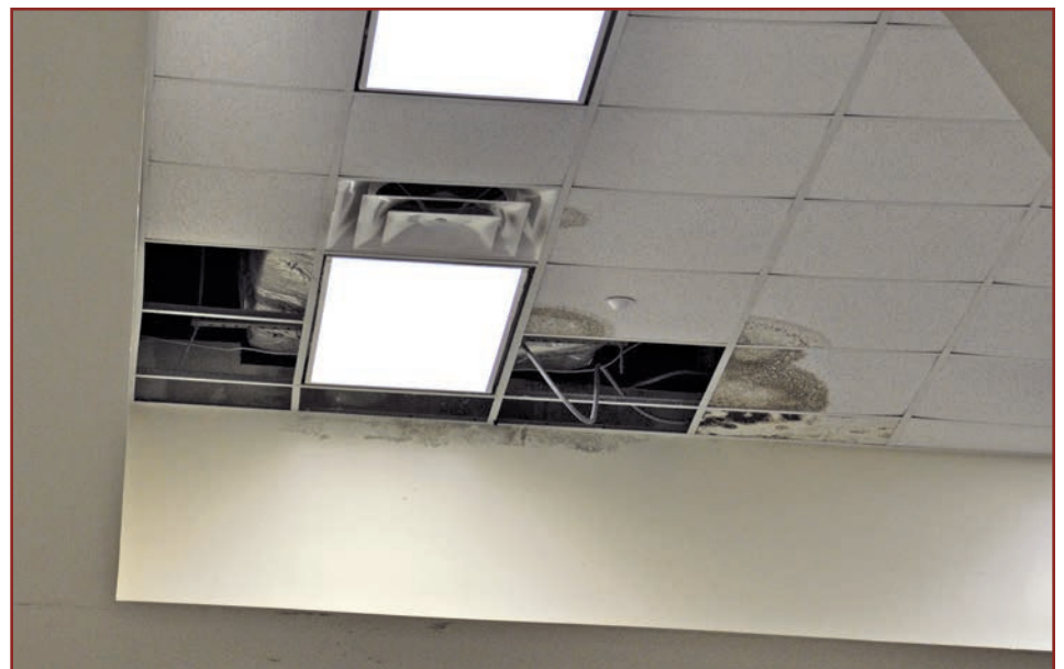
Figure 14. During Hurricane Irma (2017), relatively minor roof damage resulted in leakage that collapsed acoustical ceiling panels and wetted carpet at a school auditorium in the US Virgin Islands. Source: Federal Emergency Management Agency (FEMA) Mitigation Assessment Team.
