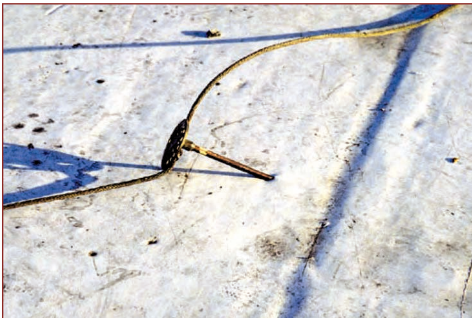
Figure 30. During Hurricane Marilyn (US Virgin Islands, 1995), a displaced air terminal punctured the roof membrane in several locations. Source: Federal Emergency Management Agency (FEMA 543). 2
