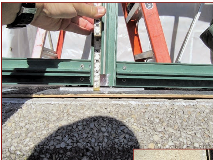
Figure 18. The portion of mullion tongue removed.
