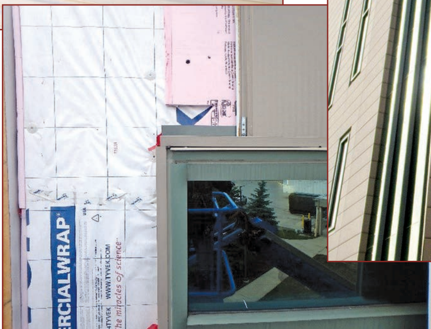
Figure 4. Panelized composite metal veneer over continuous insulation.
