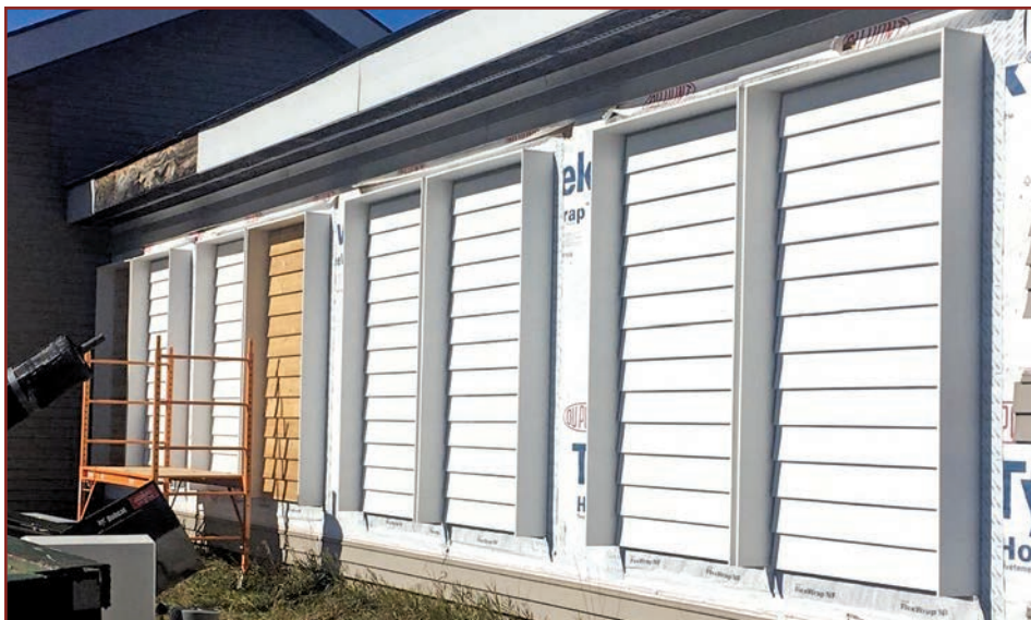
Figure 3. Exterior view of baseline walls depicting cedar siding before wall retrofits.
