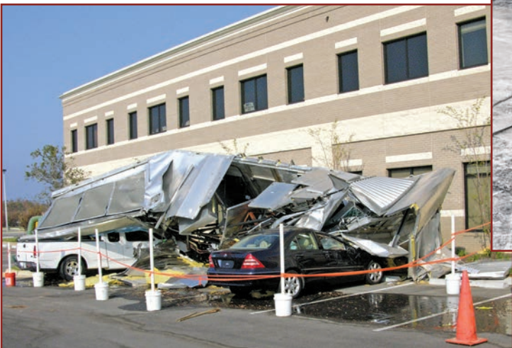
Figure 27. Although this 18,000-lb heating, ventilation, and air-conditioning unit was attached to its curb with 16 straps, the unit blew off during Hurricane Ivan (2004) because the attachment was inadequate. The Alabama medical office building was less than one year old. The estimated wind speed was 85 to 95 mph. Source: Federal Emergency Management Agency (FEMA 489). 52
