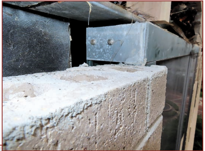
Figure 13. An end cap installed at a gap between the head and jamb and fastened in place.
