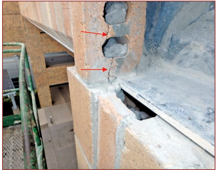
Figure 6. Vertical fractures and brick bearing less than two-thirds of the brick depth.
