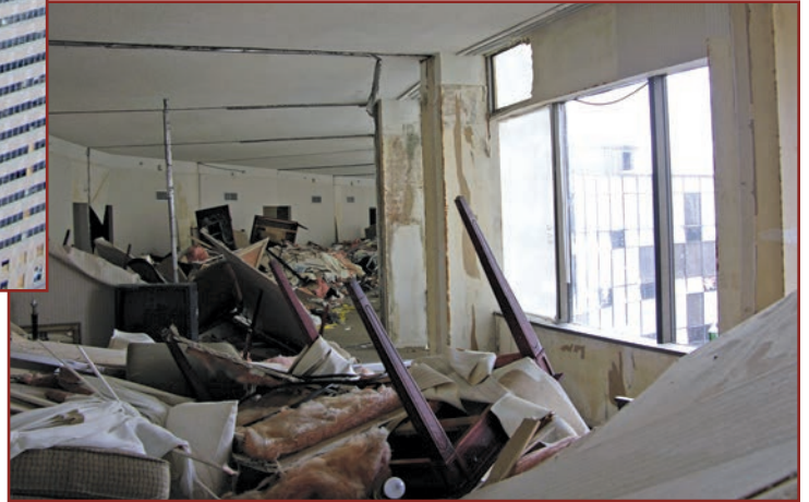
Figure 13. During Hurricane Katrina (2005), three office buildings (T1, T2, and S4) and a hotel (T3) in New Orleans had extensive glazing damage that was primarily caused by wind-borne roof aggregate. It took more than a year to replace the glazing at T1. The inset shows hotel guest rooms at T3. After the glazing was breached, development of high internal air pressure collapsed the walls between the guest rooms. The estimated wind speed was 105 mph. Source: Federal Emergency Management Agency (FEMA 549). 30
