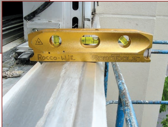
Figure 10. A pan is reverse-sloped toward the interior.
