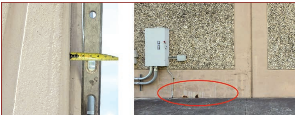
Figure 10. Extent of visible wall bowing (left) and efflorescence at crack in panel (right).
