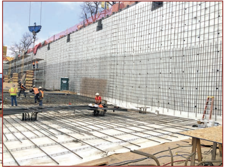
Figure 14. Reinforcing steel being installed over the top of pre-applied sheet waterproofing.
