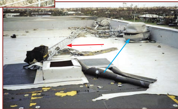
Figure 10. The collapse of the antenna tower (red arrow) at this school caused progressive peeling of the adhered single-ply membrane. Also note that the exhaust fan blew off the curb (blue arrow), but the high parapet kept it from blowing off the roof. Source: Federal Emergency Management Agency (FEMA 543). 3
