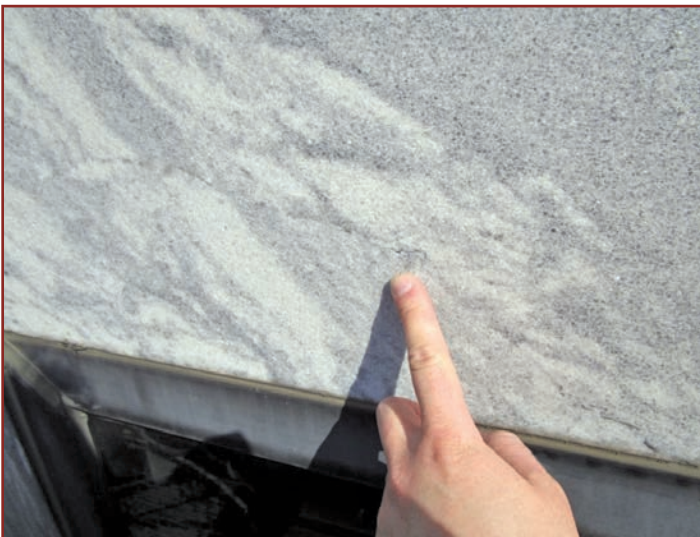
Figure 9. Typical fissure crack.
