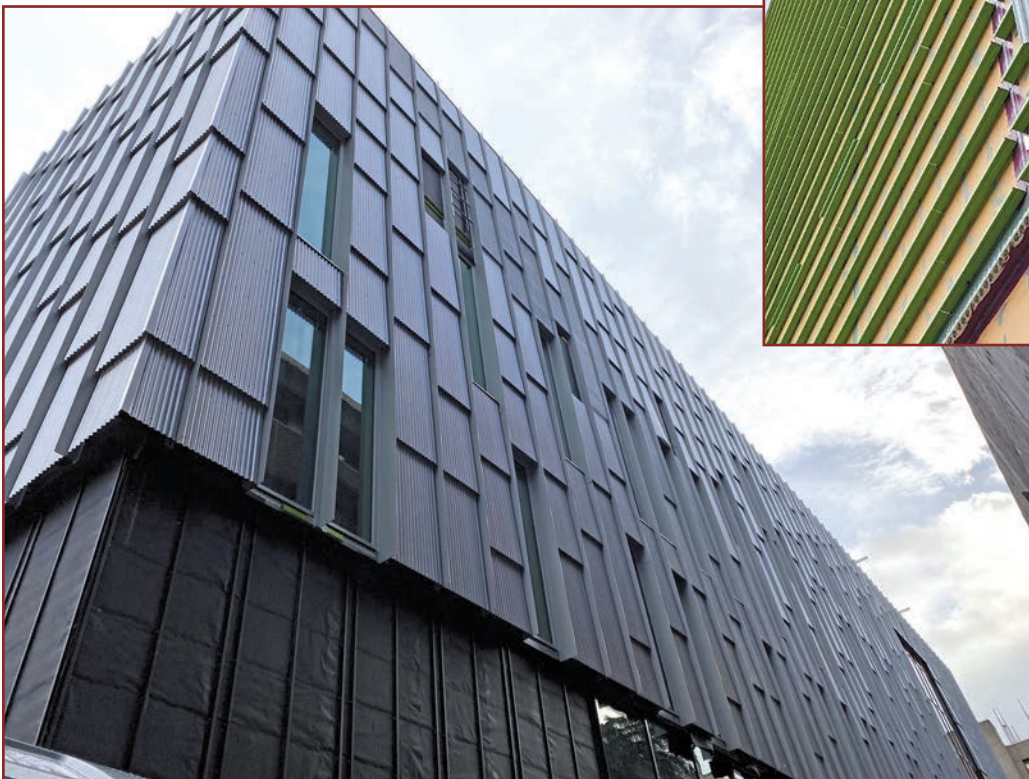
Figure 11. Panelized wall facade nearing completion.
