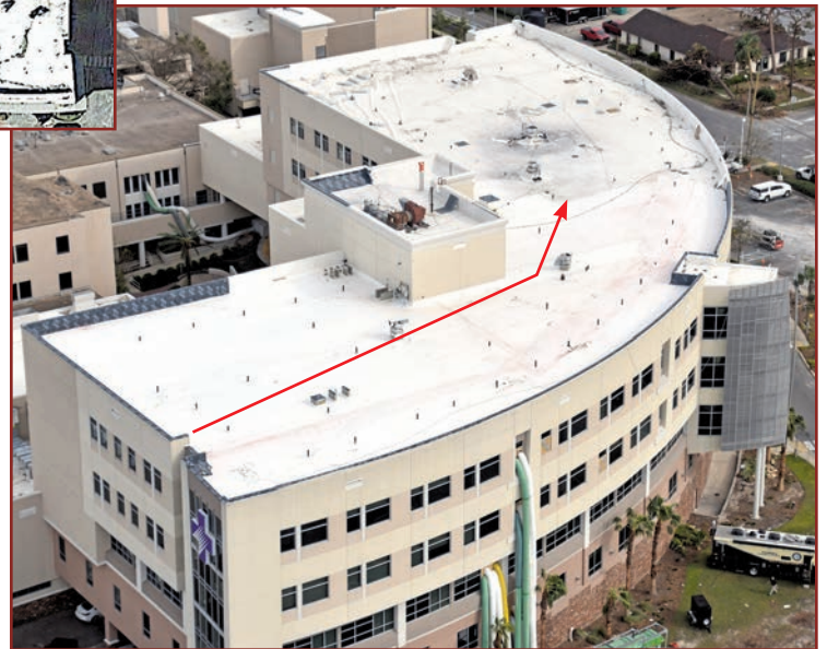
Figure 2. By the time this photo was taken, the damaged roof membrane shown in Fig. 1 had been replaced (red line). In addition to roof membrane damage, rooftop equipment and exterior insulation and finish system were blown off.
