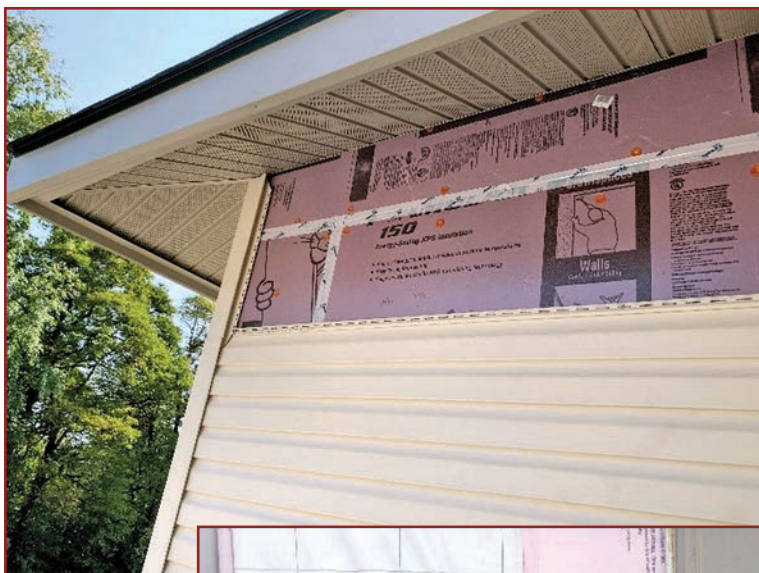
Figure 3. Vinyl lap siding veneer over continuous insulation.
