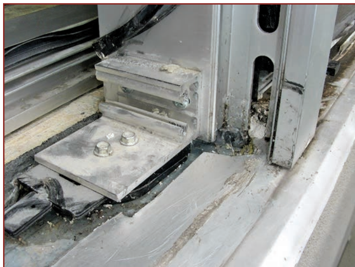
Figure 11. The back dam of the pan was cut to fit around the mullion and anchor clip.
