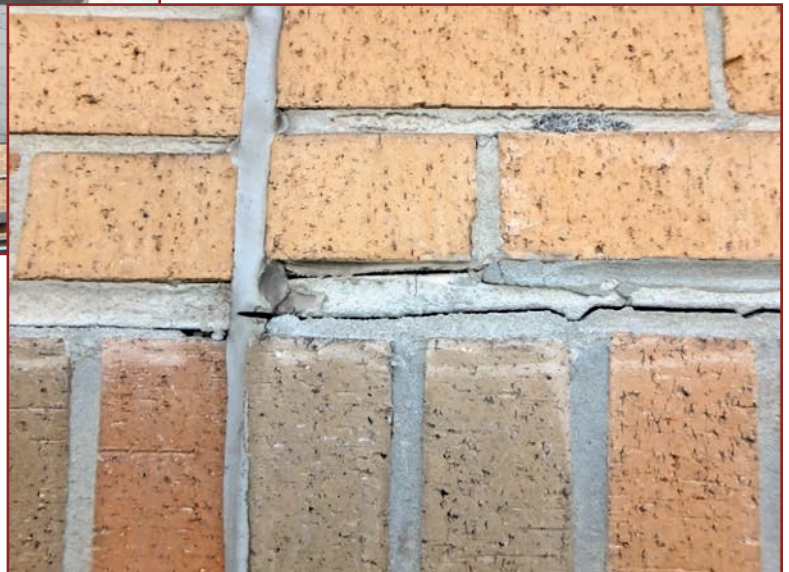
Figure 4. Typical brick mortar joint cracking.
