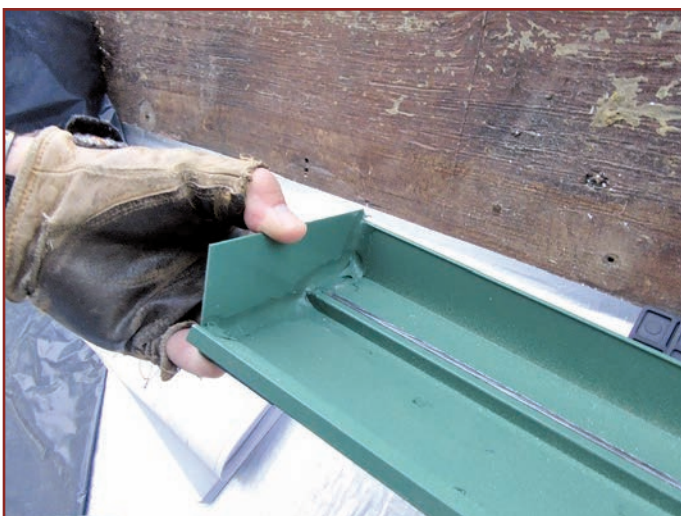
Figure 7. A subsill end dam.
