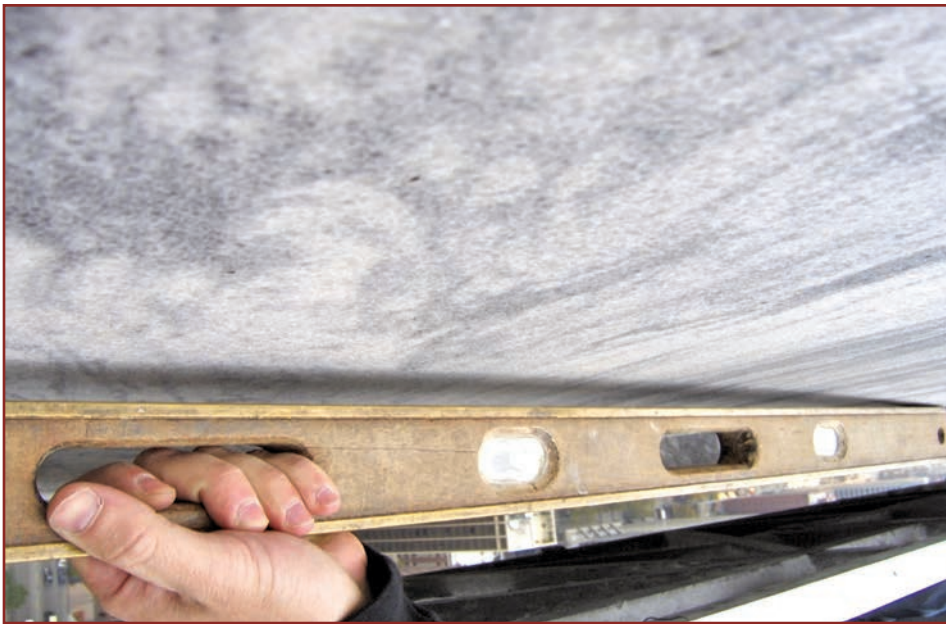
Figure 3. On-site marble bowing in relation to a straight 4 ft level.
