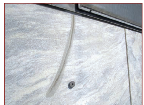
Figure 8. Typical stress crack that has been routed and sealed.
