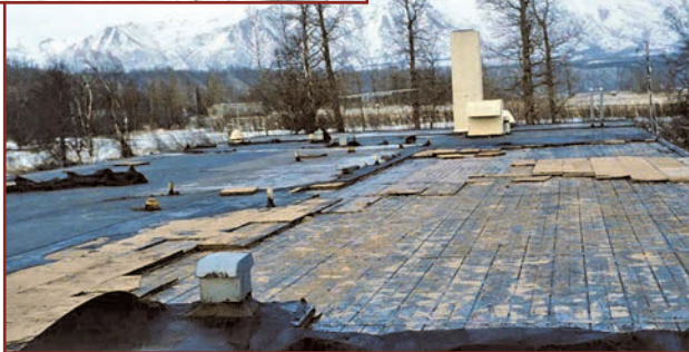
Figure 4. The roof on this school in Palmer, Alaska, blew off during cold weather in the late 1970s, thus increasing the repair costs. Membrane lifting at the edge flashing initiated the failure. The membrane was not clamped by the metal edge flashing.
