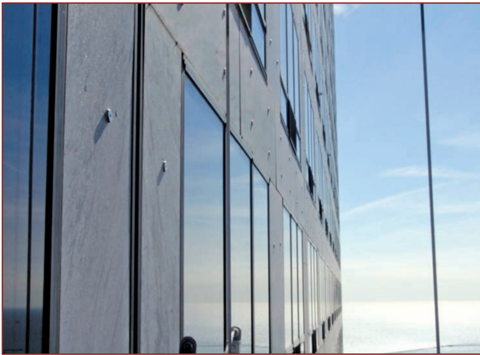
Figure 5. Overview of custom stone anchors installed on the marble facade.
