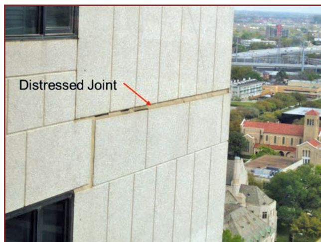
Figure 14. Apparent panel movement at a joint.
