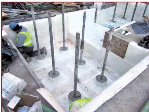
Figure 3. Rock anchor penetrations through foundation waterproofing.
