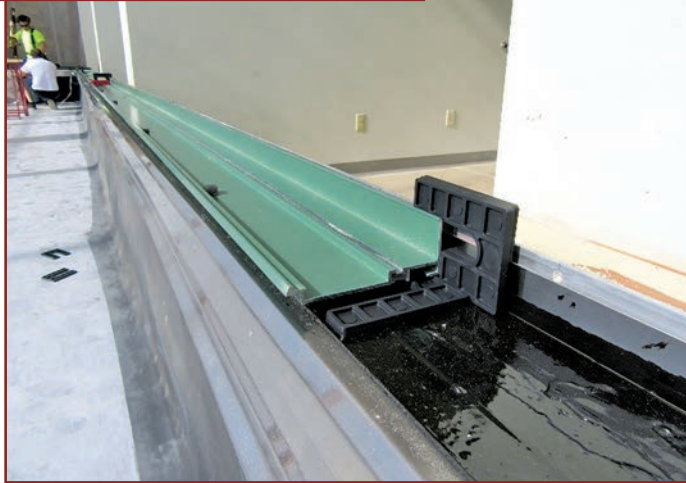
Figure 16. A subsill set and shimmed in place.
