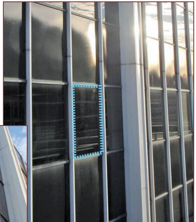
Figure 9. Representative photo of curtainwall glazing panels within the interior wind zone. The blue dashed lines frame the interior zone window analyzed in the case study.
