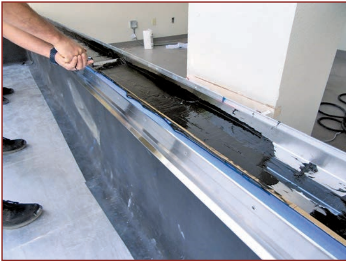
Figure 15. Fluid-applied elastomeric waterproofing troweled in place between metal flashing components.
