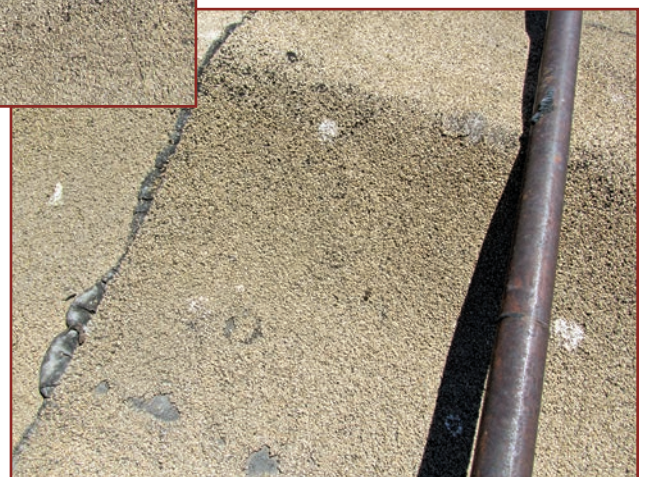
Figure 38. Progression of granule loss occurring as a result of the bird droppings.
