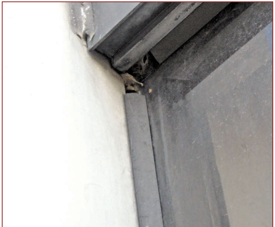
Figure 8. Example of gasket cracking deterioration in a 1965 curtainwall.
