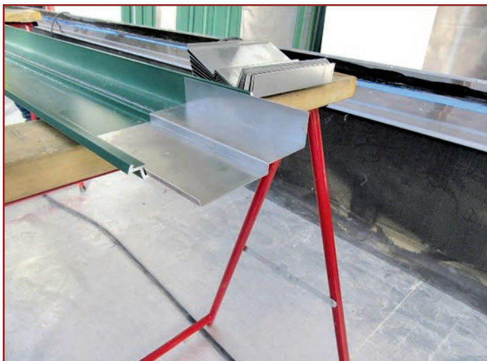
Figure 5. A subsill butt joint cover.
