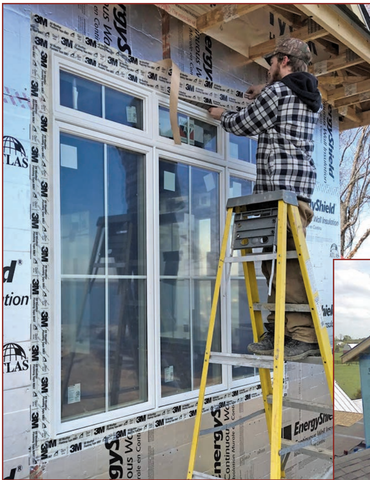
Figure 4. Adhered flashing and joint tapes used for foam plastic insulating sheathing water-resistive barrier systems and window flashing.
