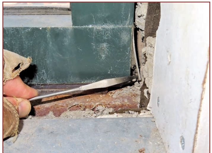
Figure 4. A loose end dam at the end of a sill.
