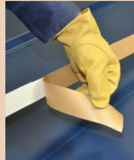
Step 4 - Remove tape/ affix to membrane
