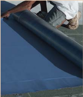
Step 1 - Install membrane
