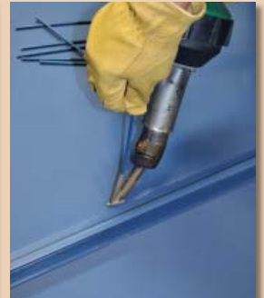
Step 5 - Permanently weld with SecureRod™
